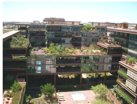
Example of buildings with landscaped decks that can screen mechanical equipment
