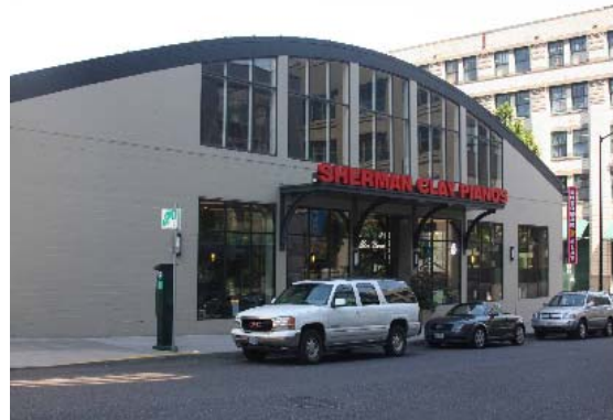
A building that contains architectural elements that visually reduce the scale of the wall
