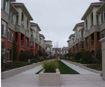
Example of Courtyard with Private Open Space, Windows Overlooking the Space
