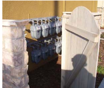
Utility equipment (i.e. meters) enclosed by a wall that is compatible with the development
