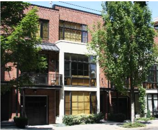
Flat roof with cornice line
