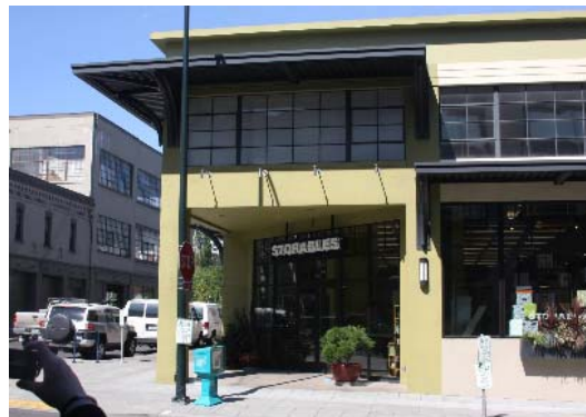
Example of a stepped roofline
