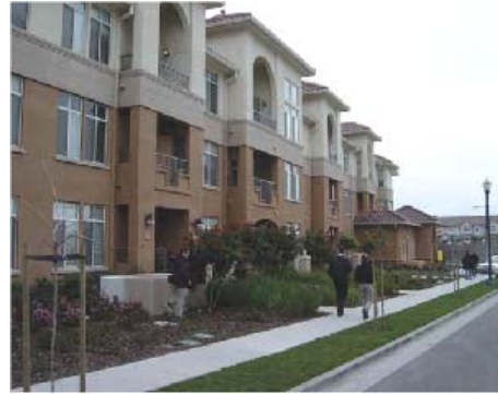
Multi-family development with extensions to the building
