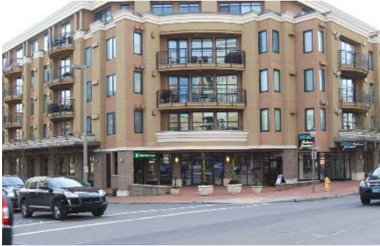
Building with a ground floor area that contains at least 50 percent in clear vision glass
