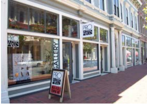
A development with glass as the predominant building material
