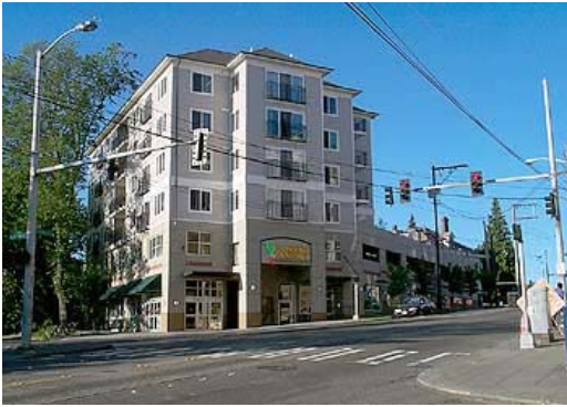
Example of a parking garage (right side) that blends into the mix-use development
